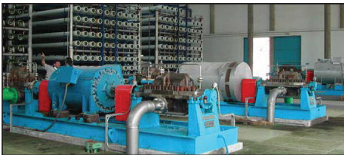
ZERON 100 Pipe work for reverse osmosis applications.
